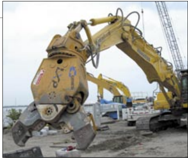
▲ A Genesis LXP being installed on the jobsite.
