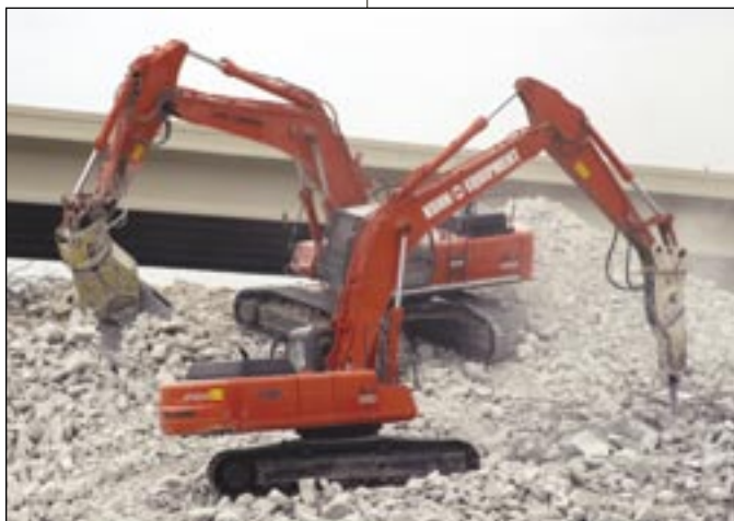
◀ Kuhn Equipment processes concrete.
